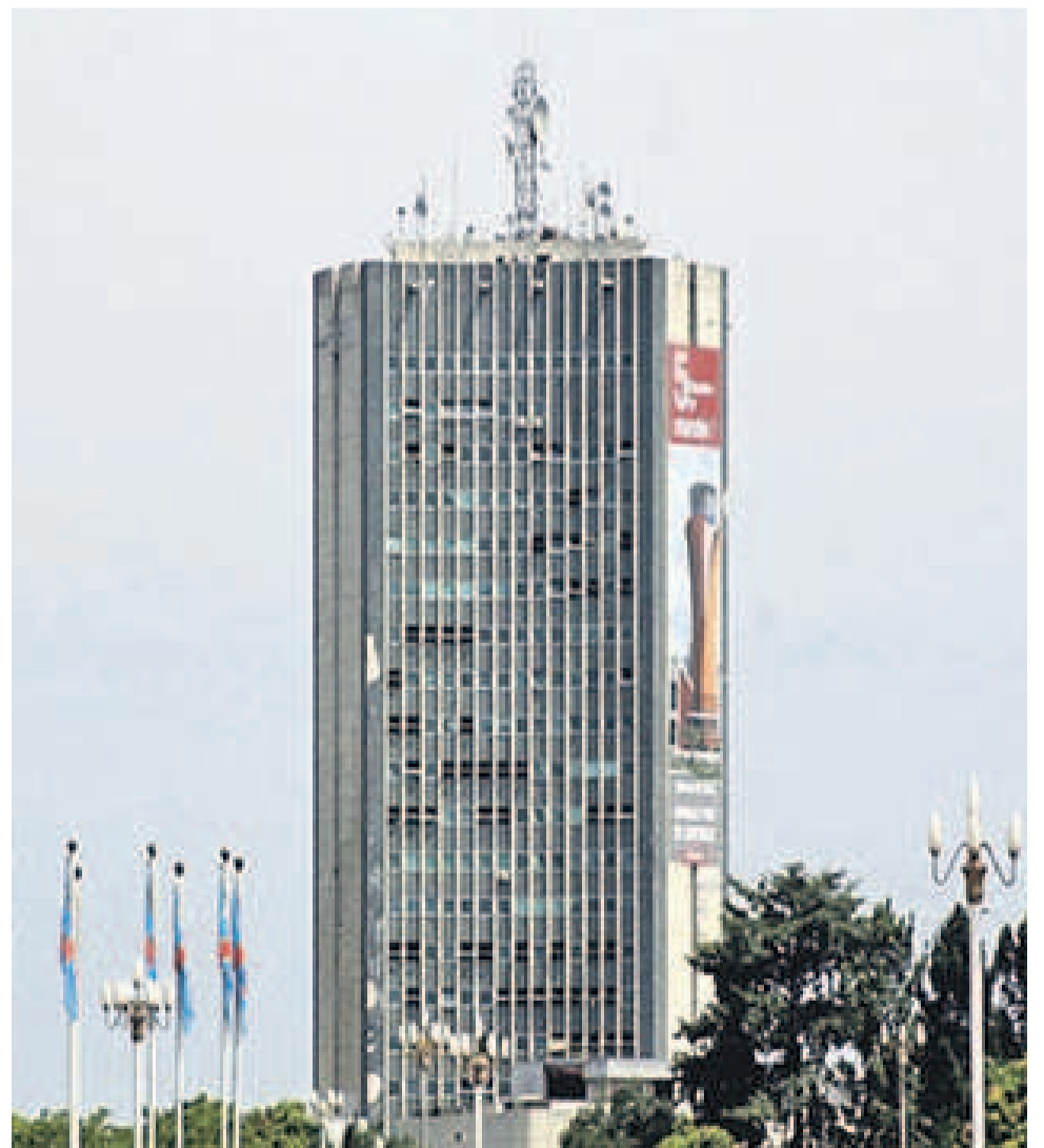
La tour administrative de la RTNC
